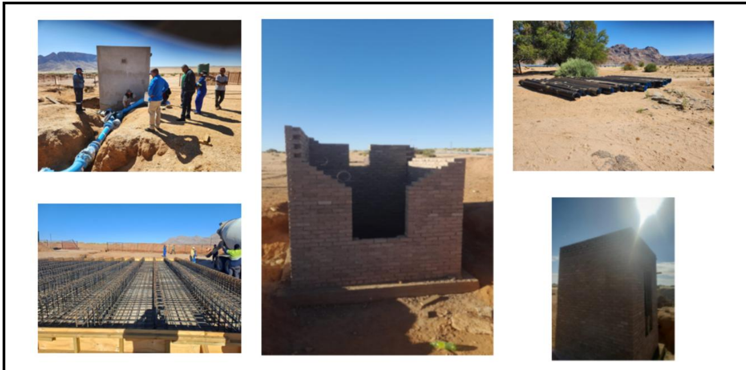
Figure 7: Pella Water Infrastructure Project 2025/2026
